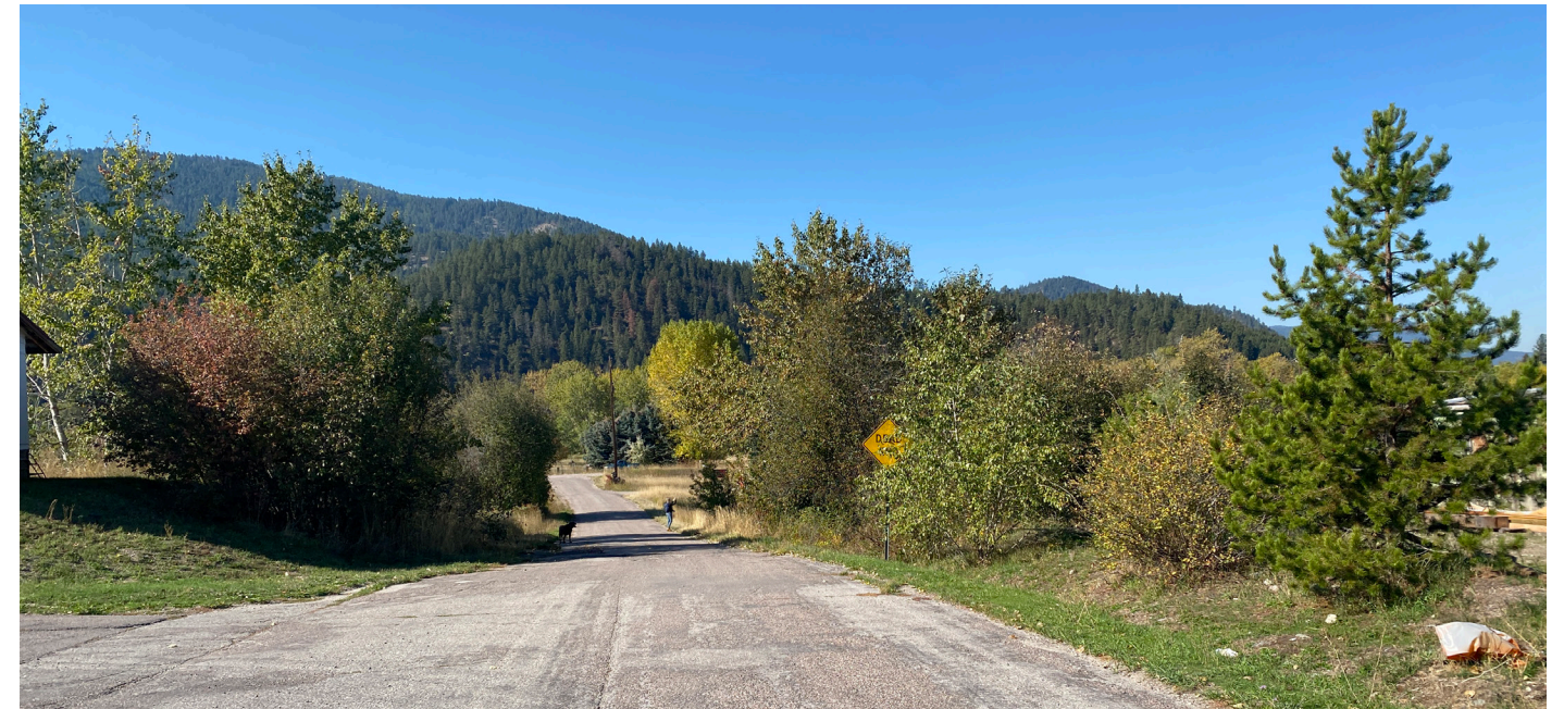
Figure 5 – Western End of Silver Street, Terminating at Clinton Community Park
